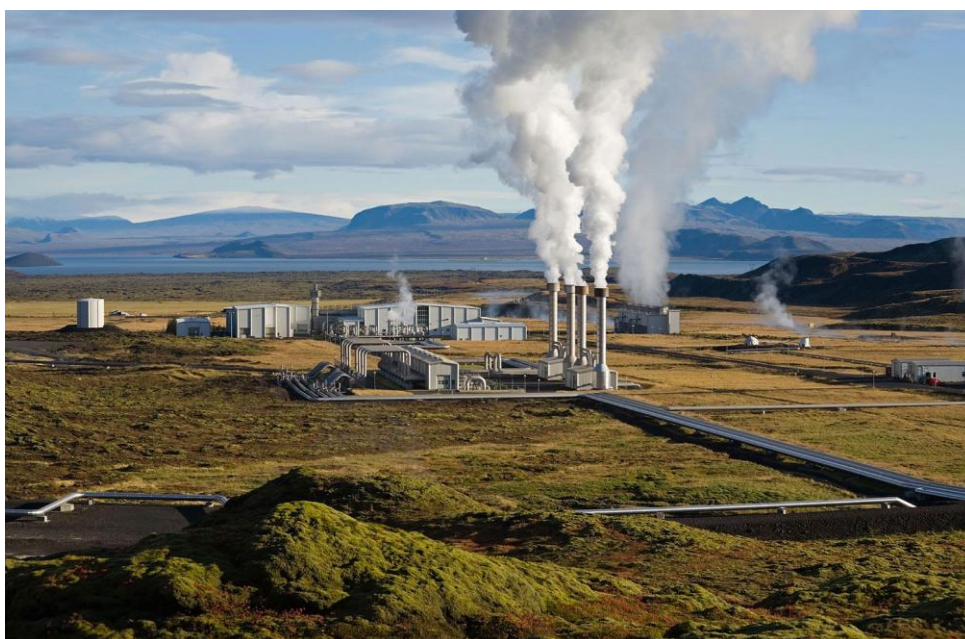
The Nesjavellir Geothermal Power Station, Iceland
